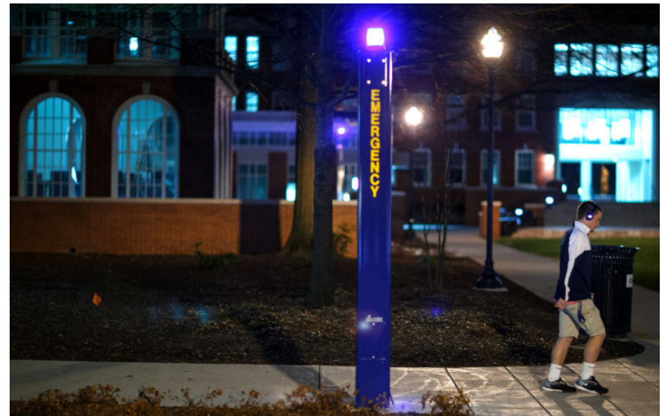
An emergency phone tower placed on a school campus Photo: Minute Man Security Technologies
