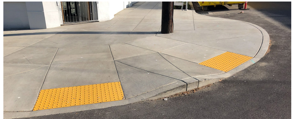
Tactile indicators are placed at the curb cuts of a crosswalk in contrasting colours. Photo: Flickr user Dylan Passmore
